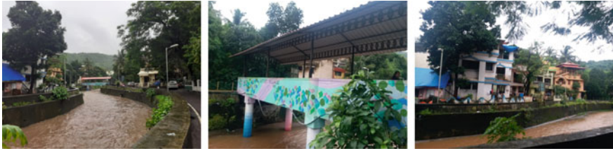
Fig. 7 Nullah or drainage canal in Artist village, Belapur. Source Authors
