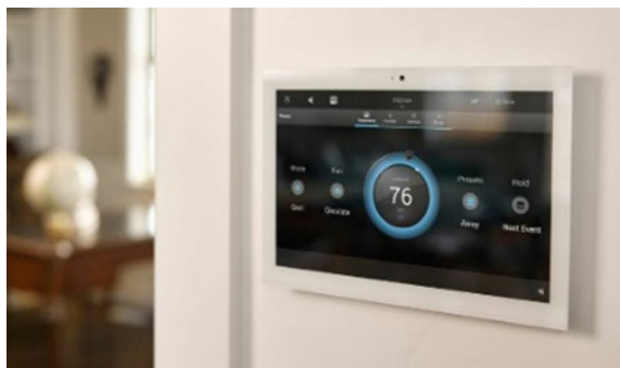
Fig. 8 Smart control panel to operate temperature of different rooms
