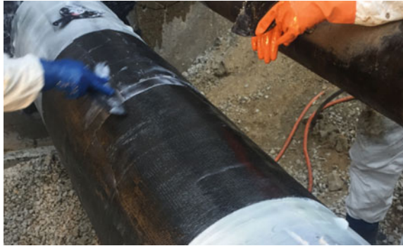
Fig. 1 Typical view of CFRP strengthening of steel pipes [1]
