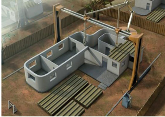
Fig. 2 Contour crafting 3D printer [12]
