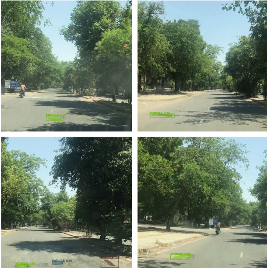
Fig. 5 Some output images from the trained Mask R-CNN model (coloured masks are the segmented potholes)
