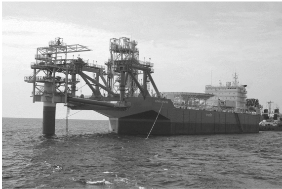
Fig. 3. Use of large-diameter bearing monopile as fixed single point mooring for the offshore industry.
