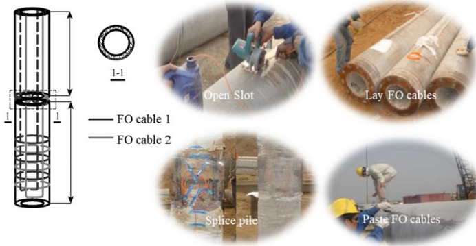
Fig. 2. Layout of FO cables on a precast pile
