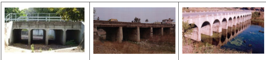
Fig. 7 Arch type BCB constructed at affordable cost
