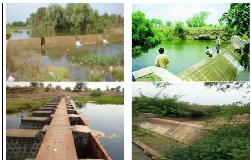
Fig. 3 Typical cement plugs
