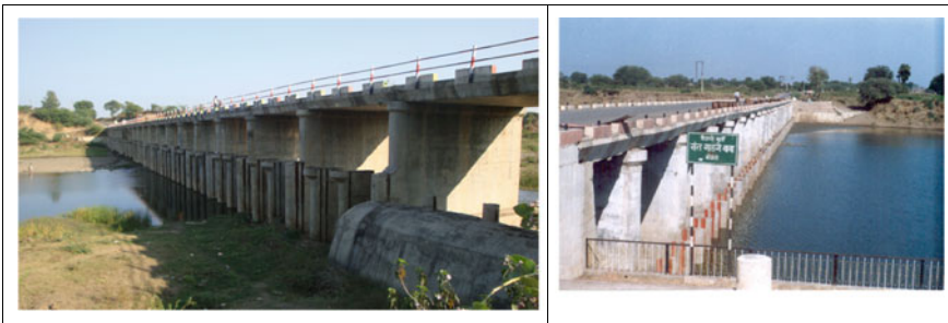
Fig. 2 Bridge cum Bandhara on Purna River, T. Daryapur
