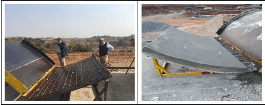
Fig. 10 Formwork and mold
