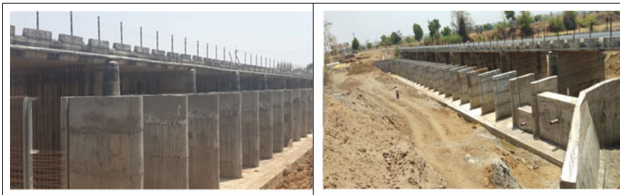
Fig. 12 Bridge cum Bandhara across Andhari River
