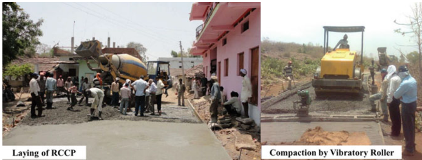
Fig. 2 RCCP trial length being constructed under Pilot Project Package No. MP-0511 [36]
