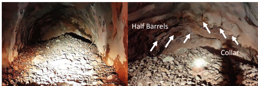
Fig. 5 ESD 001 first trial (4580-ESD-001 new 51 mm drill plan—G_5.0 × 5.0_51 bit, chainage 37.3 m)
