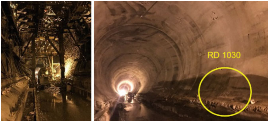
Fig. 25 Final lining of tunnel in critical zone
