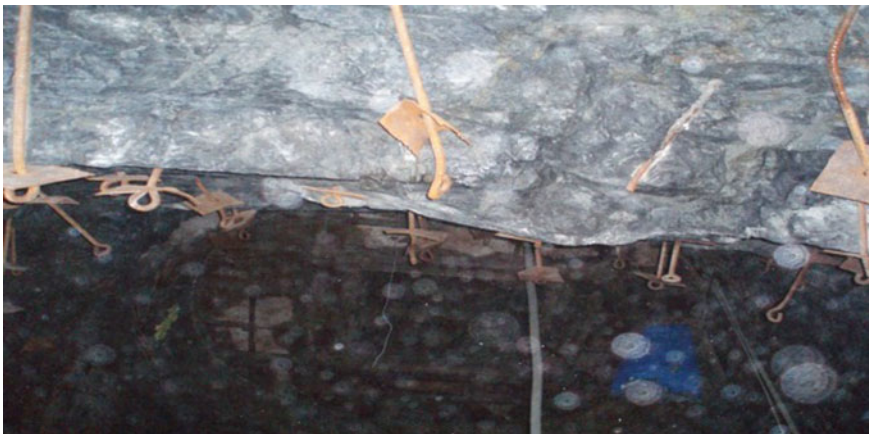
Fig. 8 Roof of the excavation at 206 m
