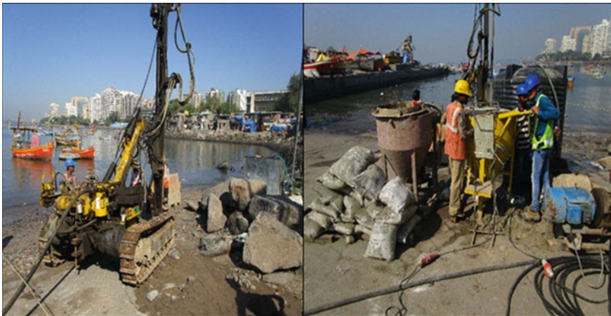
Fig. 8 Drilling of holes (Left) and Grouting of holes (Right)
