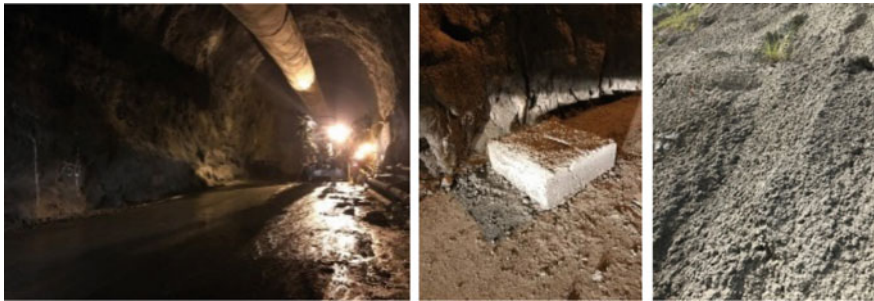
Fig. 2 Concrete structures built in underground tunnel, cavern and in surface
