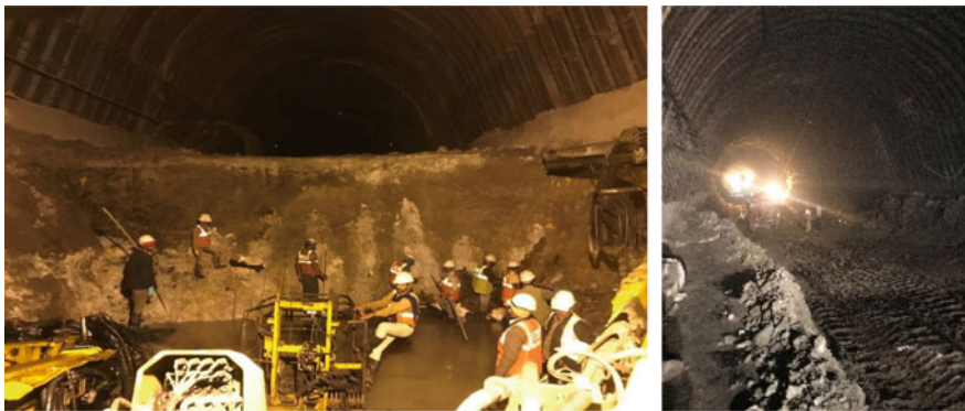
Fig. 9 Benching in stages
