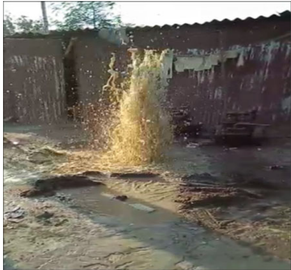
Fig. 9 Pressurized muddy water during drilling of grout holes
