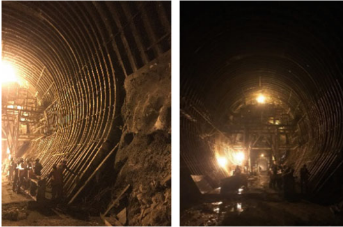
Fig. 24 Support extended to invert level along with horizontal struts
