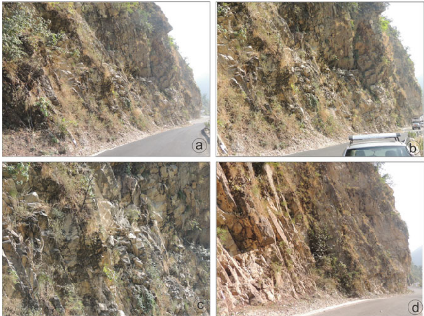
Fig. 3 Rockmass conditions of the cut-slope in the study area
