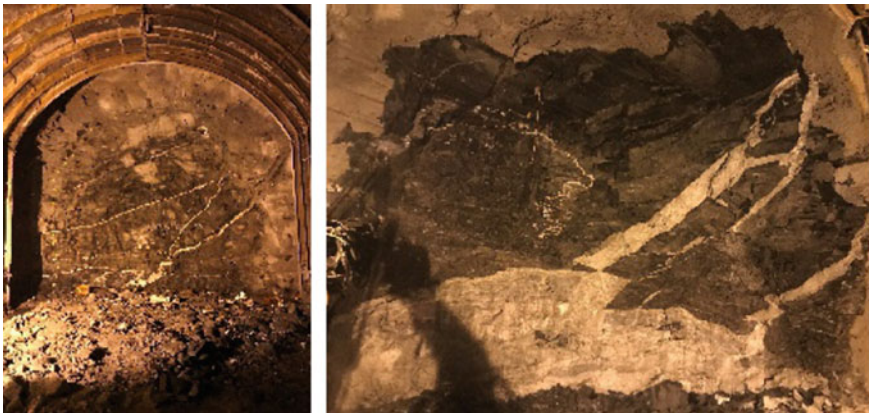
Fig. 3 Varying geological condition encountered after every blast
