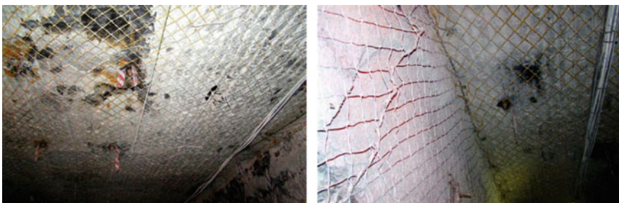
Fig. 30 Installed roof nets at the mine
