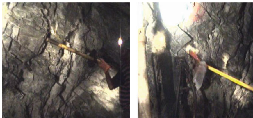
Fig. 25 Photos of mechanical “jaws” in underground operation
