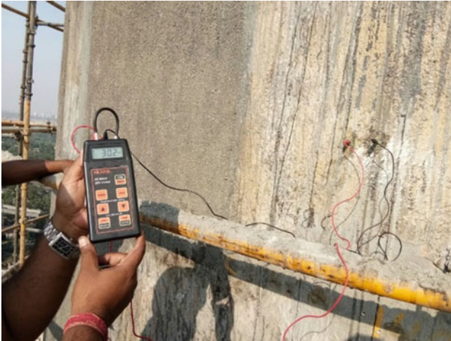
Fig. 19.15 Humidity meter to measure moisture content on RCC Chimney
