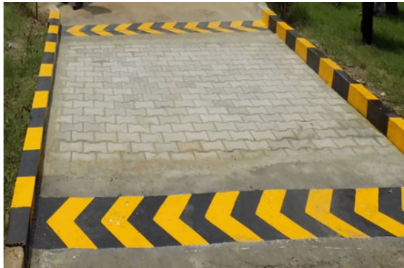
Fig. 10.3 Flyash based geopolymer concrete block road stretch
