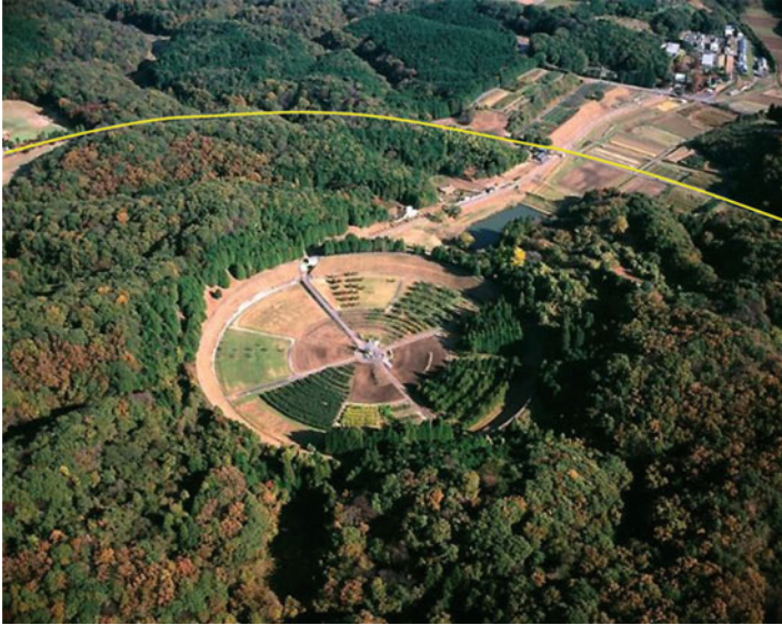
Fig. 12.1 Gamma Field of IRB (Courtesy of IRB, NARO). Yellow line: Restricted area
