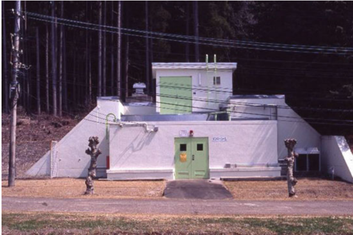
Fig. 12.3 A shielded building of the Gamma Room inside the restricted area. (The photo taken by the author with the permission of IRB, NARO)
