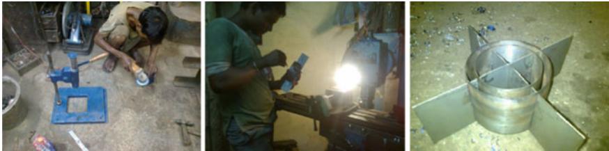
Fig. 7 Fabrication of different components
