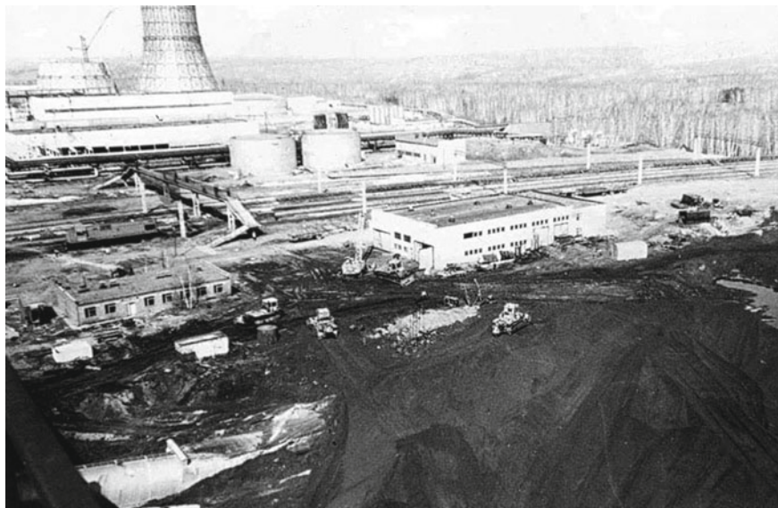
Fig. 1 Coal pipeline “Belovo-Novosibirsk”, Belovo, Kemerovo Region, Russia
