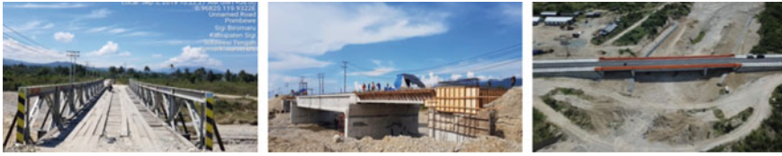
Fig. 2 Pre-during-post rehabilitation and reconstruction stage
