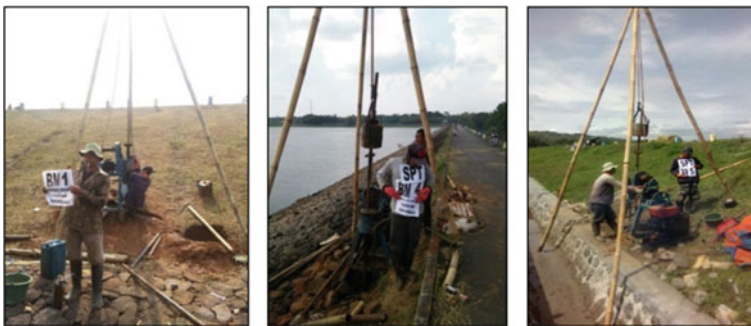
Fig. 2 Boring at Klego Dam
