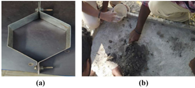
Fig. 1 a Paver block mould. b Mixing of materials
