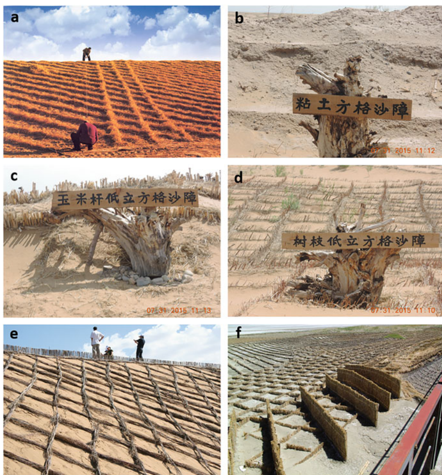
Fig. 8.8 Wheat straw (a), clay (b), cotton straw (c), corn straw (d), willow twig (e), and reed (f) checkerboard sand barriers (a, e, f from Wang 2011; b, c, d provided by Xian Xue)
