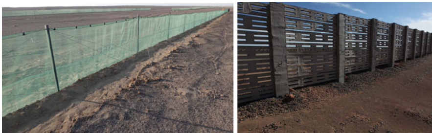
Fig. 8.1 Sand-blocking fences with different porosities and heights (Photos courtesy of Yanping Yu and Tao Wang)
