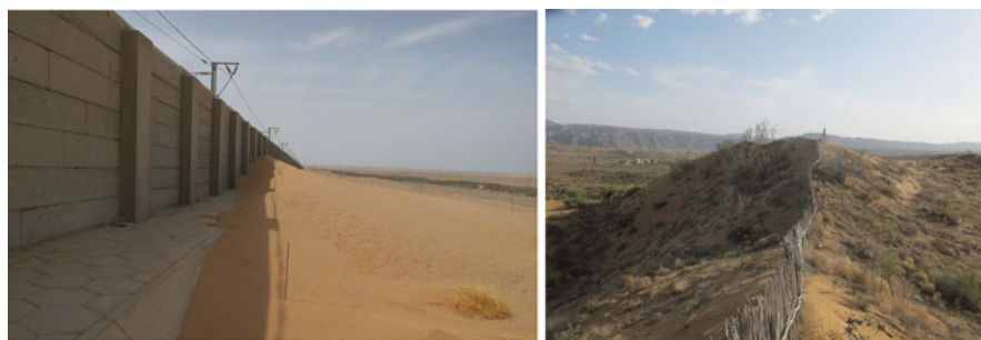
Fig. 8.2 Windbreak wall (left) and sand-prevention dike (right) (Photos courtesy of Tao Wang and Zishan An)
