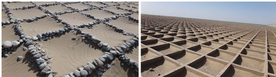
Fig. 8.4 Gravel and clay checkerboard sand barriers on the Qinghai-Tibetan Plateau (Photos courtesy of Yanping Yu)
