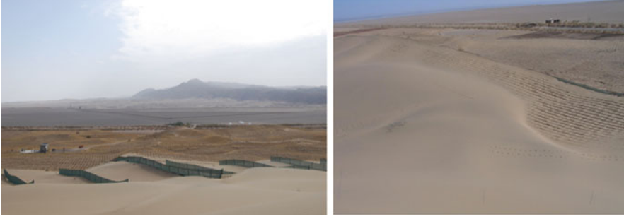
Fig. 10.7 Upright sand-blocking fences and semiupright sand-fixing wheat-straw checkerboard barriers on the eastern margin of Mingsha Mountain (provided by WM Zhang)
