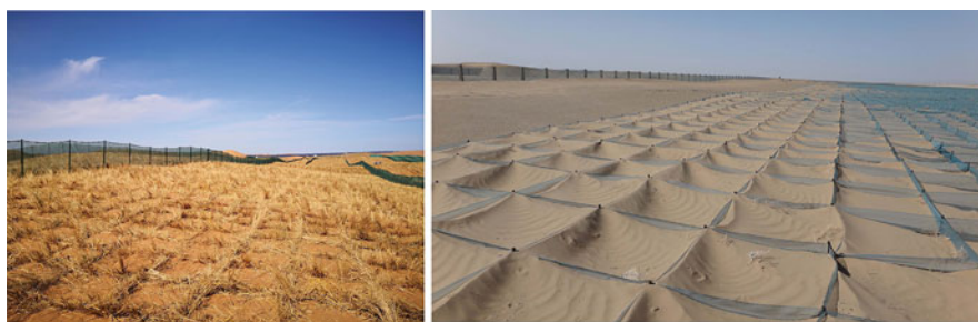
Fig. 8.3 A checkerboard barrier at the preliminary stage and at the mature stage with a concave face (Photos courtesy of Yang Gao and Yanping Yu)
