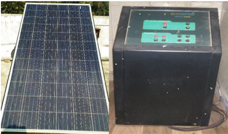
Fig. 2 Solar PV panel with converter
