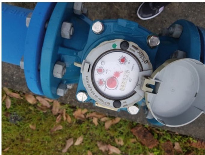
Fig. 37.2 Bulk meter capsule reading
