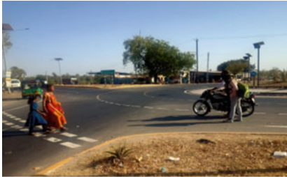
B2 Lack of road safety control devices
