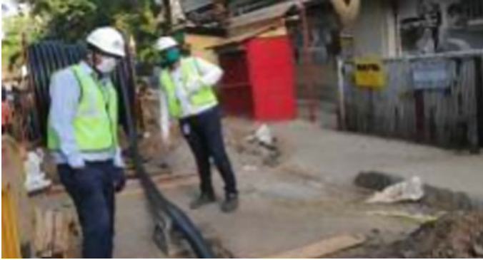
Fig. 13 Cable pulling using winch machine
