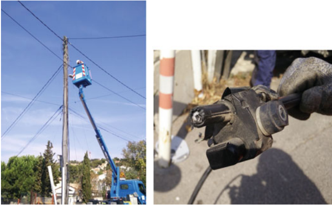
Fig. 3 Illustration of neutral break detected by AMI system
