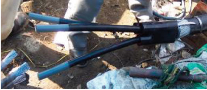
Picture 2 Water barrier components incorporated in cable jointing kit
