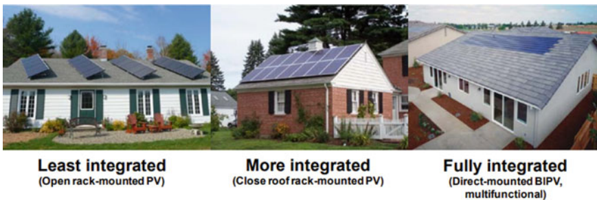
Fig. 1 Integration of BIPV panel in a residential rooftop Source Building energy 2011, DOE 2011 [1]
