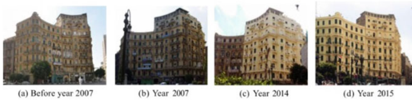
Fig. 2 Example of an exterior limestone cladding coated with a self-cleaning coating that resists algae growth (c) and (d) [9]
