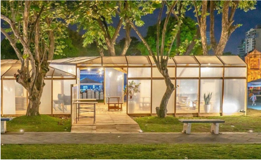
Fig. 10 The emergency quarantine facility (EQF) (Source WTA Architecture and Design Studio, 2020)
