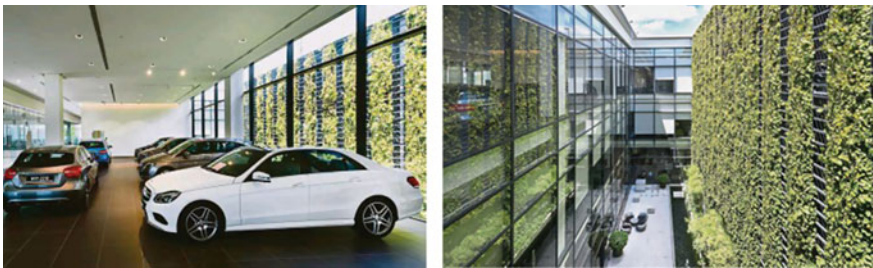
Fig. 4 Mercedes Benz showroom at Balakong featuring glass facades and courtyards as elements of sustainable design
