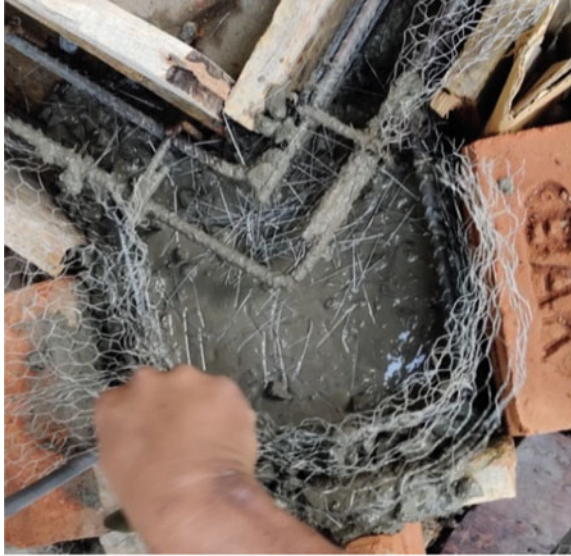
Fig. 3 RC frame joint with steel fibre
