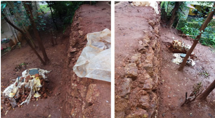
Fig. 7 Two views of the completed wall built using TGSB technology
