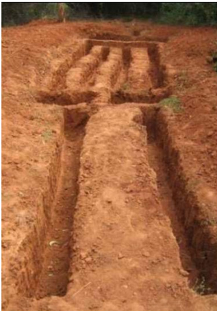
Fig. 3 Making of SHEFROL ® channels and tanks excavating soil
