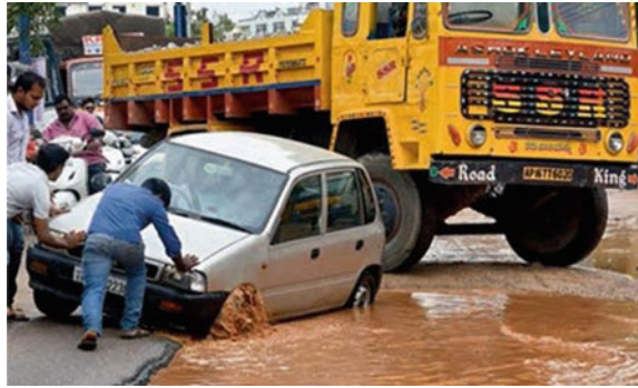
Fig. 1 Road accidents due to potholes
