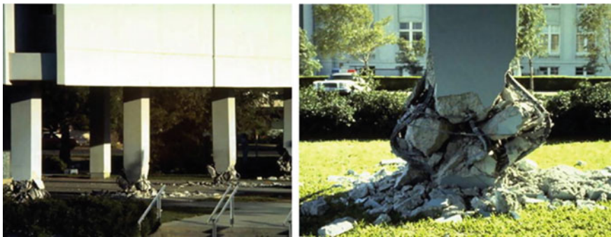
Fig. 1 Plastic hinges in Imperial Valley Services Building during the 1979 Imperial Valley Earthquake [2]
