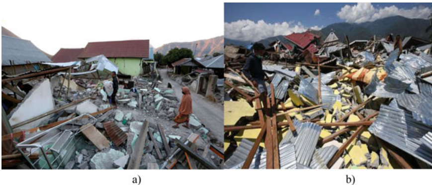
Fig. 1 The collapse of houses under; a Lombok Earthquake 2018 [6], and b Palu Earthquake 2018 [7]
