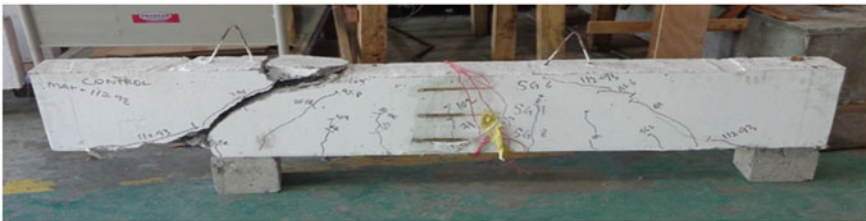
Fig. 6 Failure mode of the control beam
