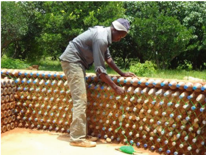
Fig. 3 Supporting material: cross-shaped cable (green wires) [31]
