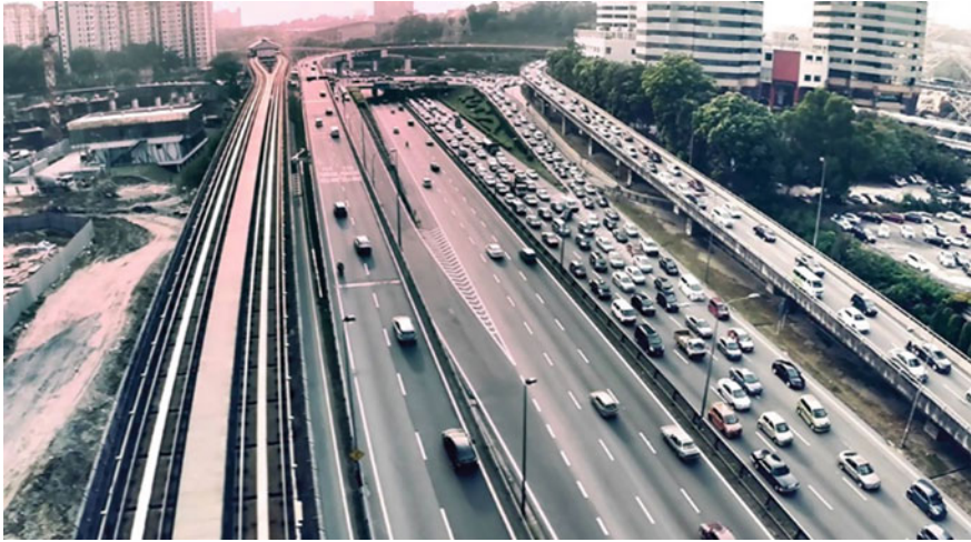
Fig. 1 An overview of the Route FT02 Federal Highway [3]
