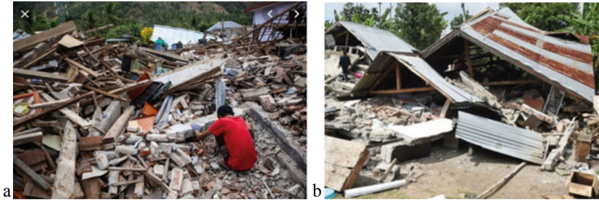
Fig. 9 Brick masonry collapsed in Lombok 2018 a full collapsed ( https://nasional.kompas.com ); b wall collapsed ( https://tirto.id )
