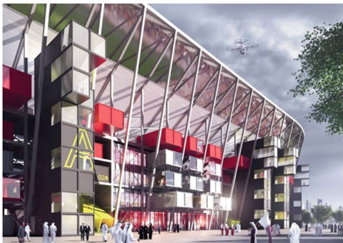
Fig. 11 Shipping Containers for Temporary Ras Abu About Stadium, Qatar FIFA World Cup 2022 [25]
