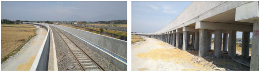
Fig. 1 Application of the PSSV structure of Adi Soemarmo Airport Railway Track
