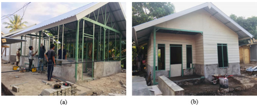
Fig. 2 The application of RISBA in Lombok (Lombok Post-Earthquake 2018)
