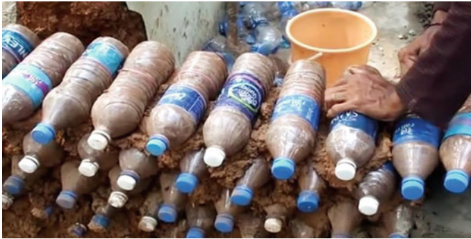
Fig. 4 Sand filled plastic bottle bricks [33]
