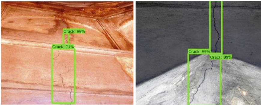
Fig. 7 Detected defects—crack
