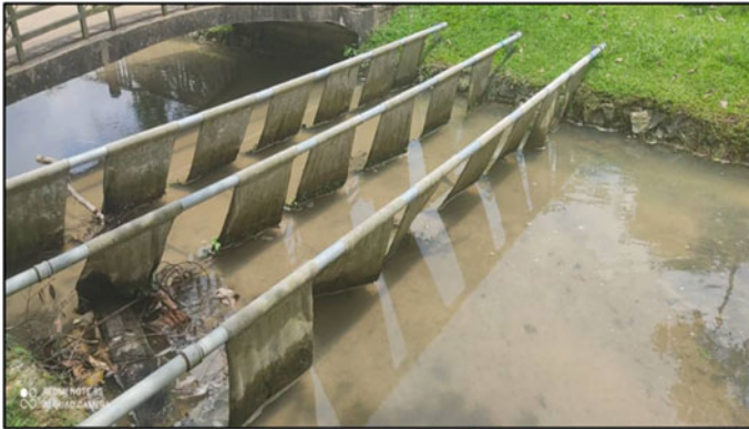
Fig. 2 Material arrangement at the site
