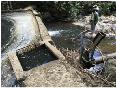
Reservoir dam and intake
