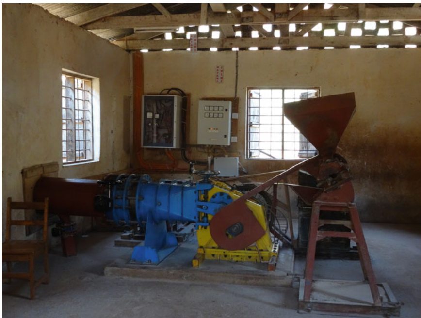
Fig. 9 Power generation infrastructure along with the milling machine
