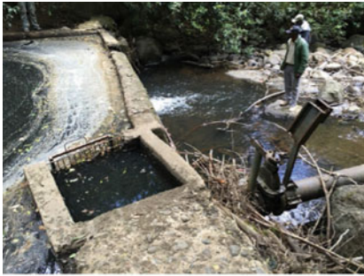
Reservoir dam and intake
