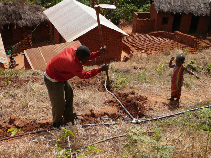
Fig. 7 A man burying the pipeline in the ground
