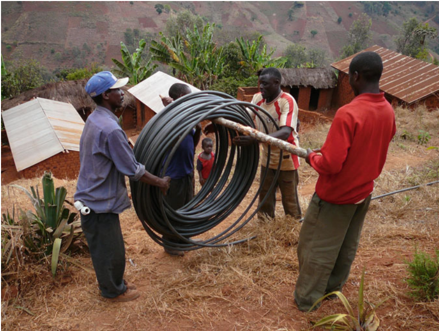
Fig. 6 Villagers installing branch pipelines
