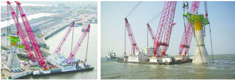
Fig. 3. Installation of wind turbines on Thornton Bank, Belgium [7].
