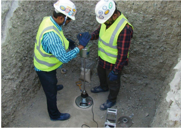
Fig. 4. Trial pit reveals the competent materials beneath the oil tank foundation.
