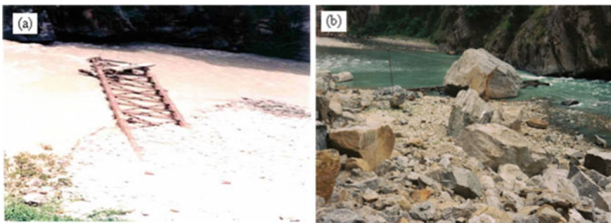
Fig. 8.8 a A bridge fallen in the Bhagirathi River near Dabrani after June, 1978 ‘D.M. Landslide and Flashflood’ b another bridge covered by rocks after November, 2004 Landslide
