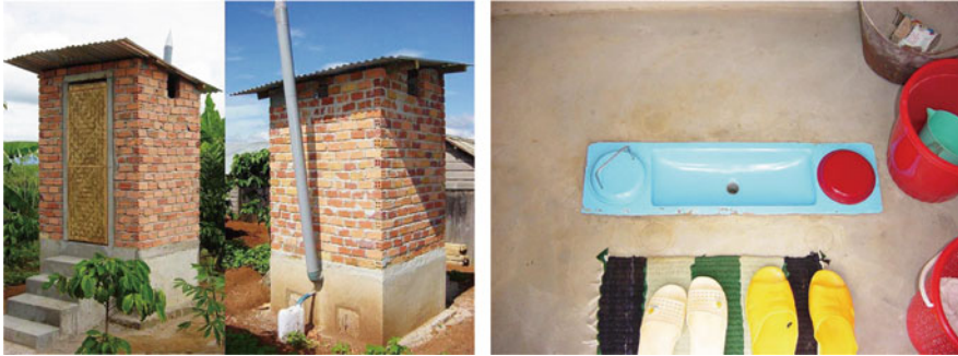
Fig. 12.2 A UDDT in the case of Vietnam: (left) outside views of a UDDT; (right) inner view of a UDDT. (Adapted from Harada and Fujii 2020)
