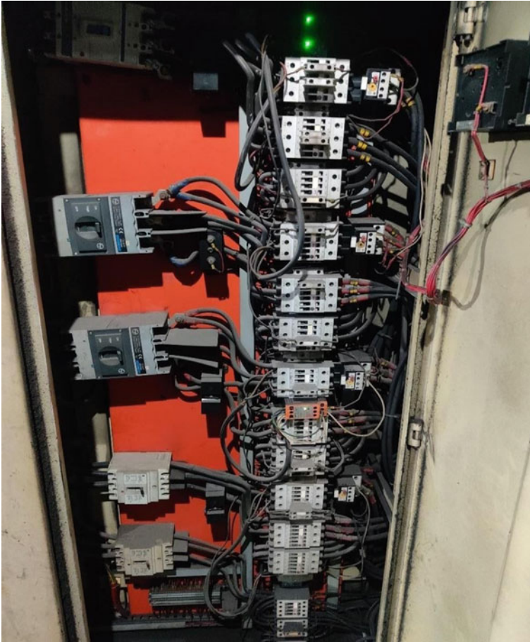
Fig. 4 Connections in star delta method with contactors and timers
