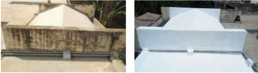
(a) Unpainted Roof
