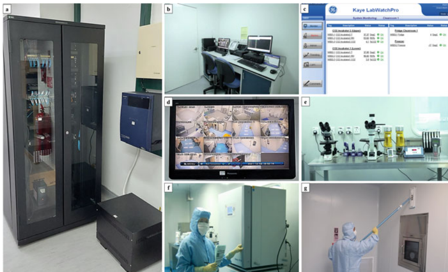
Fig. 3.4 cGMP Facility Management and Monitoring in CTERM, UKM. (a–c) Building and equipment monitoring system; (d) CCTV security camera; (e) Equipment for environmental monitoring (air sampler and particle counter); (f) Equipment maintenance and service by authorised personnel; (g) Facility personnel cleaning
