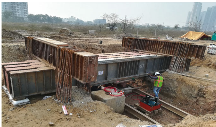
Fig. 4 Anchored reaction beam setup
