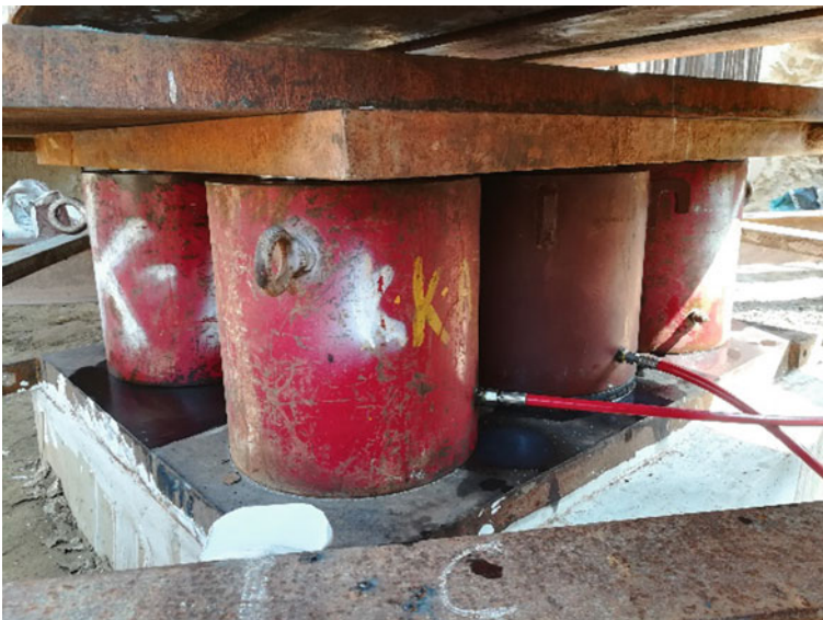
Fig. 6 Hydraulic jack configuration
