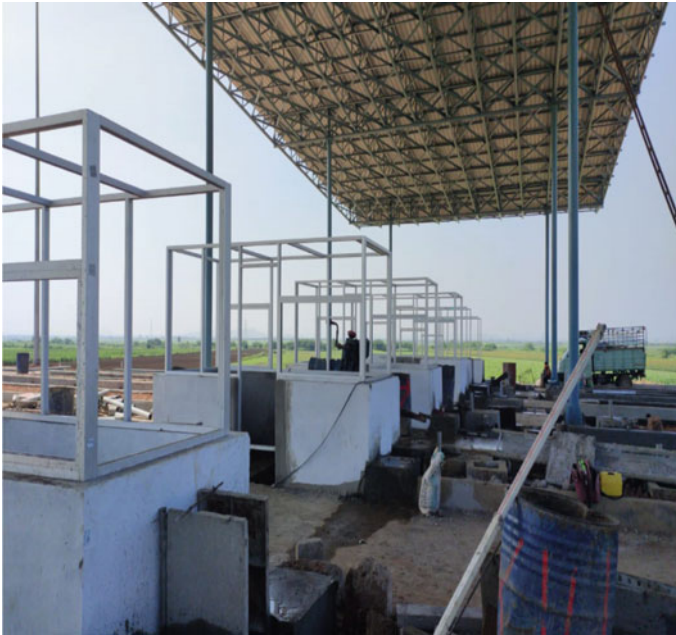
Fig. 5 Cabins in toll plaza
