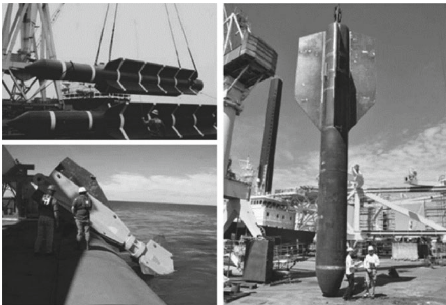
Fig. 2 Different Variations of DPAs. (Top Left) Torpedo Anchor with conical tip, (Right) Torpedo Anchor with parabolic tip and (Bottom Left) OMNI-Max anchor (Randolph and Gourvenec 2011)
