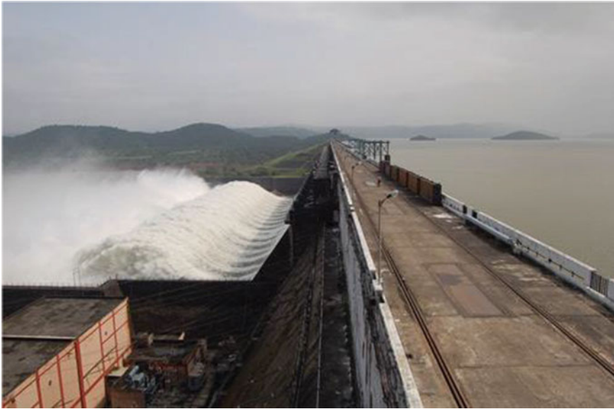
Fig. 2 Picture of Ukai dam. Source guj-nwrws.gujarat.gov.in
