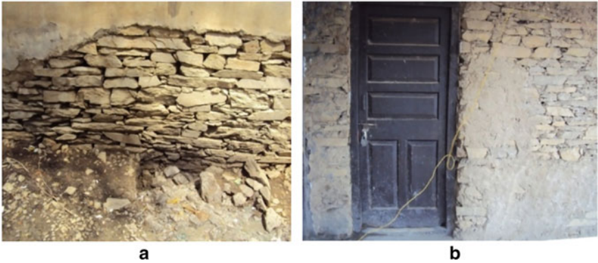
Fig. 6 a Dry rubble stone masonry, b Dry rubble stone masonry
