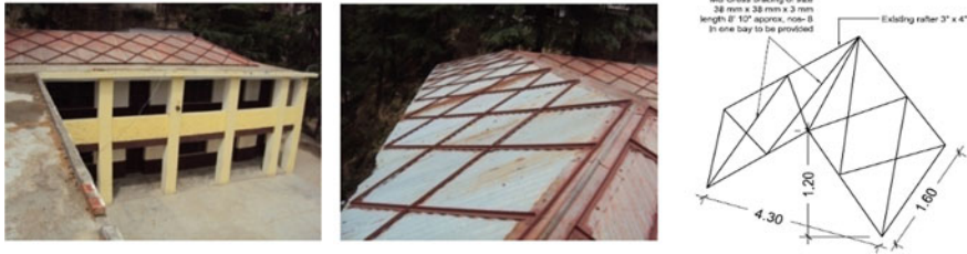
Fig. 15 Cross-bracing in wooden roof truss
