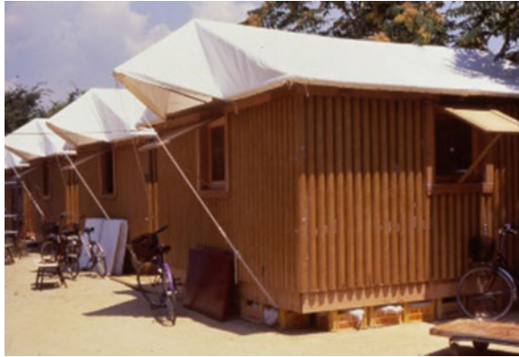
Fig. 8 Cardboard shelters. Courtesy Paper log house Kobe. Takanobu Sakuma
