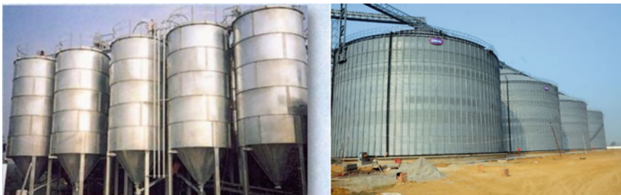
Fig. 9.14 Commercial hopper bottom and flat bottom storage silos
