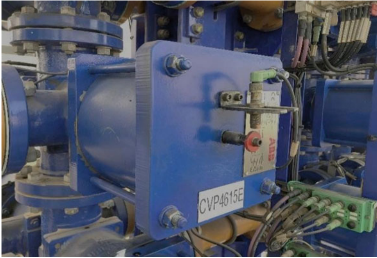
Fig. 4 Manifold valve with added sensor
