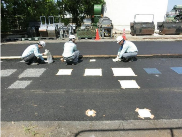
Fig. 3 Installation of modeled delaminations
