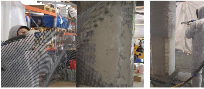
Fig. 8 Strengthening of a column with spraying method
