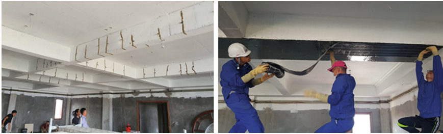
Fig. 1 Strengthening of cracked RC beams using CFRP sheets
