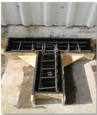
(a) Steel cage in wooden mould
