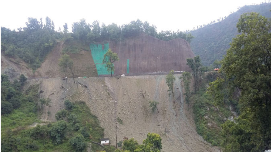
Photograph 7 Dumping of excavated material on downhill slope
