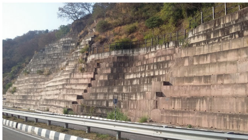
Photograph 3 Probable stabilization measures for steep cut slopes
