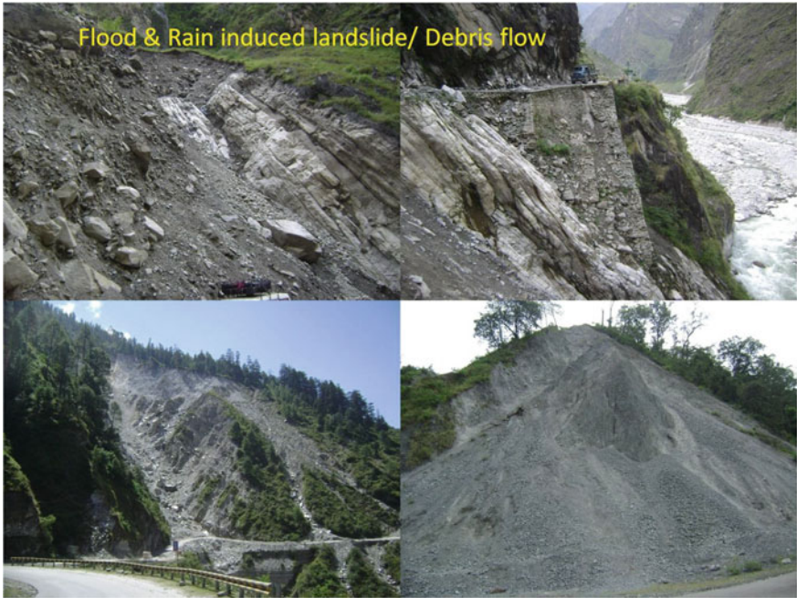
Photograph 2 Highway breached and many new landslides occurred on NH-58
