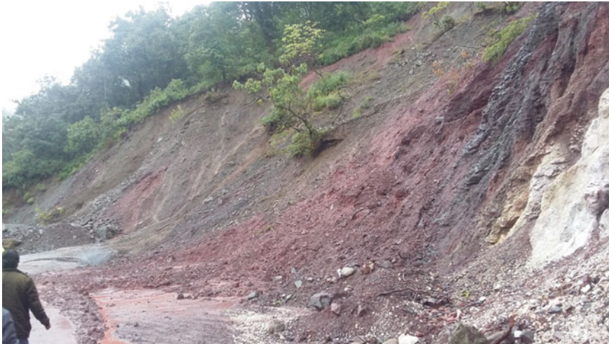
Photograph 5 Condition of the failed cut slope on widening portion of highway
