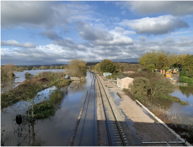
Fig. 1 A flooded turnout. The picture courtesy of East Midlands Railways
