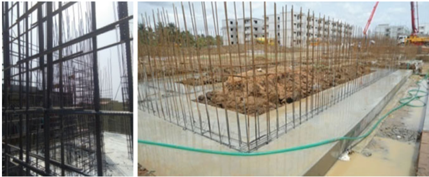
Fig. 1 Wall reinforcement
