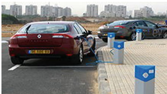
Fig. 7 Renault EV charging stations
