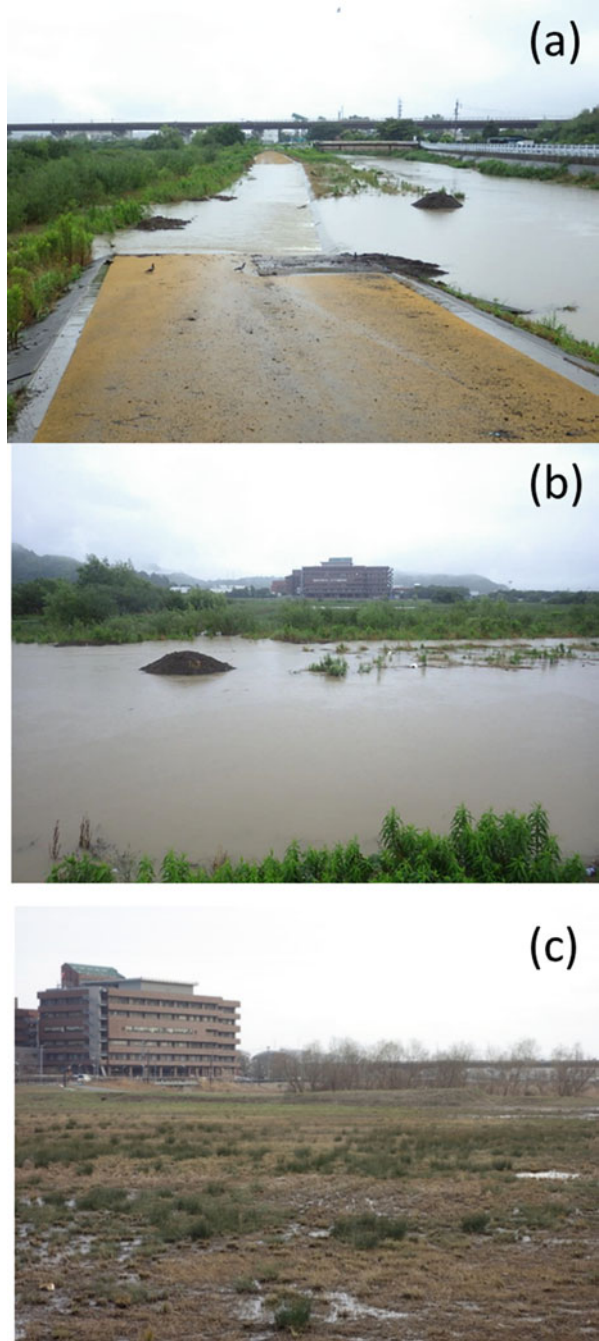
Fig. 14.1 The functioning Asahata flood control basin. (a) Floodwaters overflowing part of the levee (overflow dike), entering the FCB. (b) FCB during floods. (c) FCB under normal circumstances
