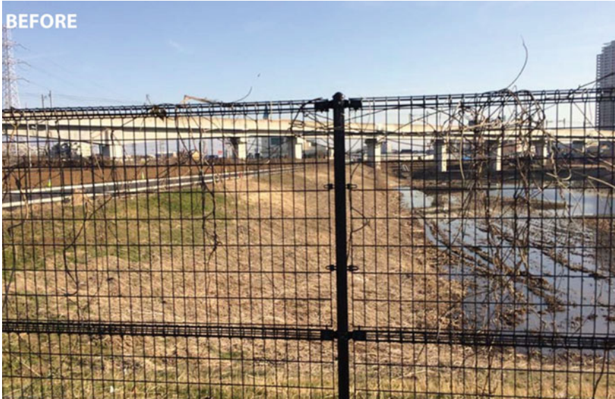
Fig. 15.6 Retention pond prior to redesign (Nikken Sekkei Ltd.)
