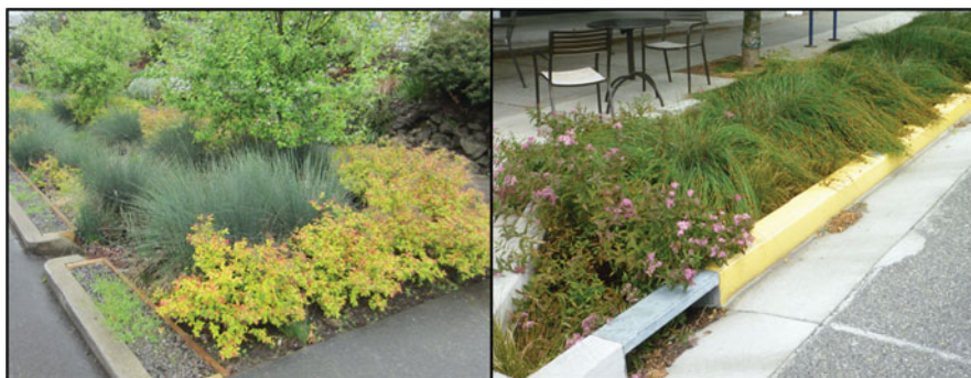
Fig. 18.2 Bioswales. These features capture stormwater and filter out pollutants (Source: City of Portland)
