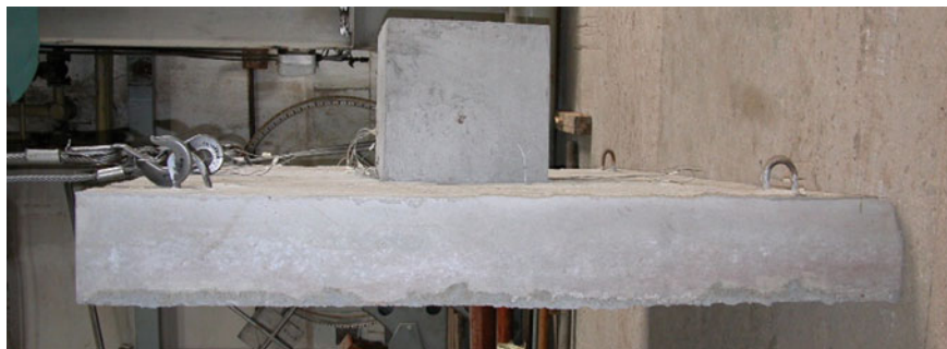
Fig. 2 Prototype in [7] after punching failure. Side view
