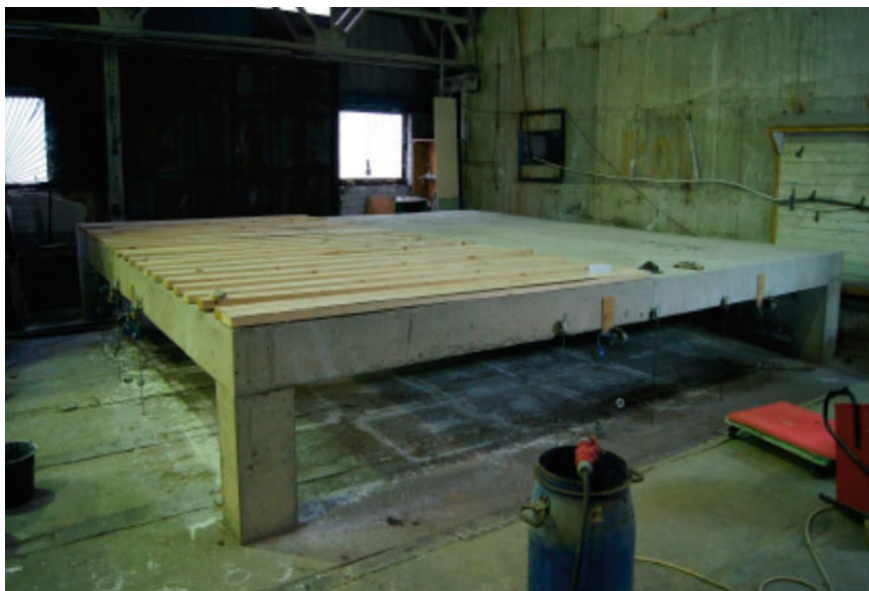
Fig. 3 General view of the prototype after concreting
