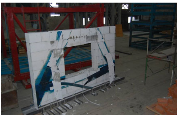
Fig. 8 General view of carbon-reinforced prototype wall after testing
