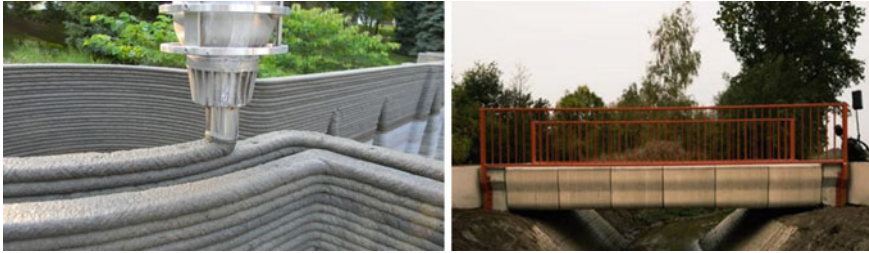
Fig. 2 3DCP using concrete mix: (a) Rudenko [9], (b) Salet, TU/e [10]
